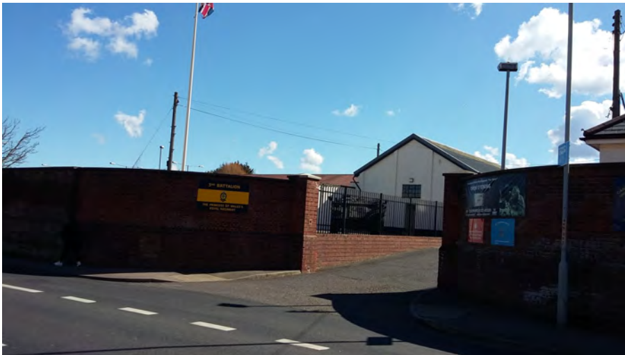
The present Barracks site
